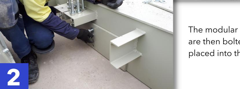
The modular weighbridge pieces are then bolted together and placed into the subframe.
